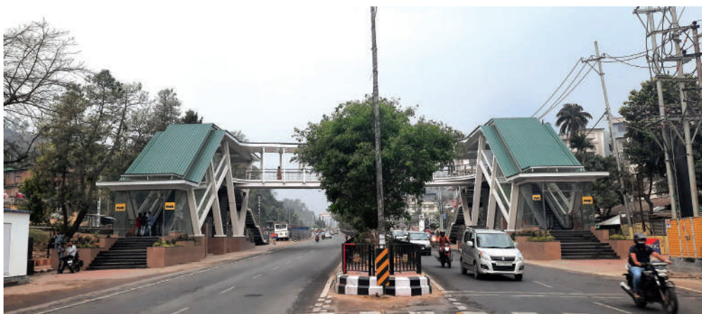
Kamakhya Gate Foot Over Bridge, Guwahati
